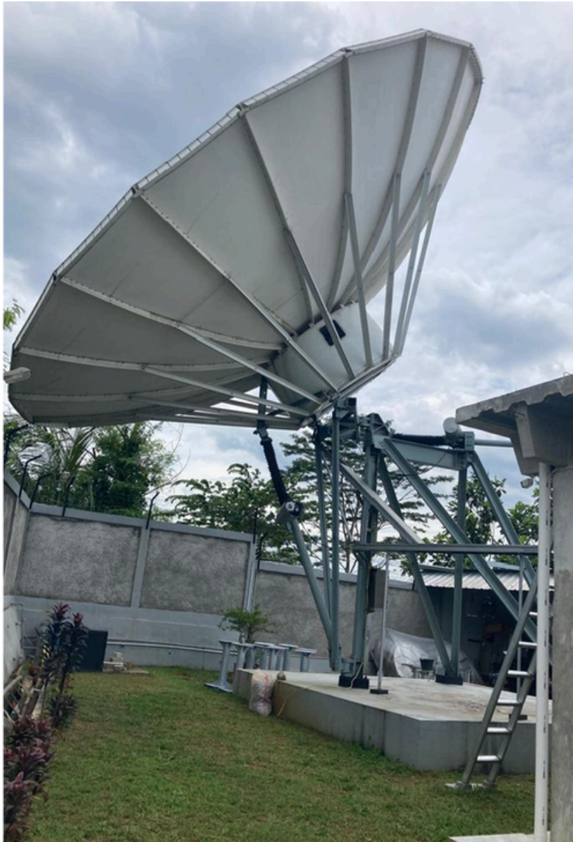
Antenna C- band 9.3m
