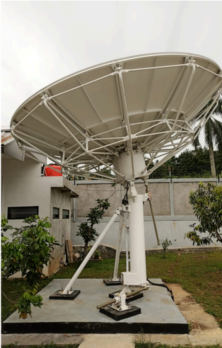
Antenna Ku- band 4.5m
