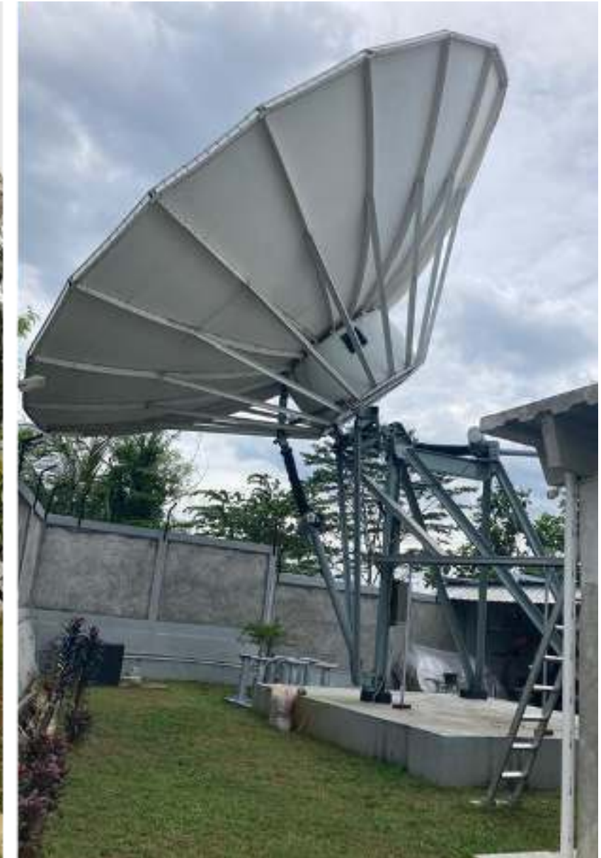
Antenna C- band 9.3m
