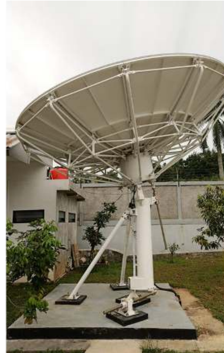
Antenna Ku- band 4.5m
